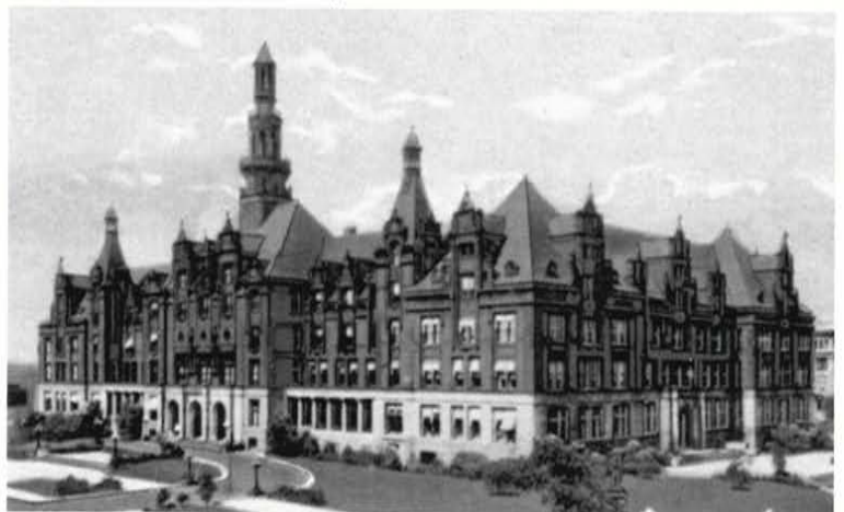
St. Louis City Hall was built in 1894. The 90-ft. center tower and two smaller towers were removed in 1936 because of corrosion.
