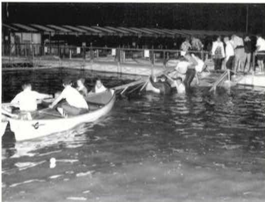
In September 1968 a bridge holding over 50 Maritz people and spouses collapsed at Tan-Tar-A Resort in Missouri during a creative conference. Nobody was seriously injured, but it was a frightening experience.
