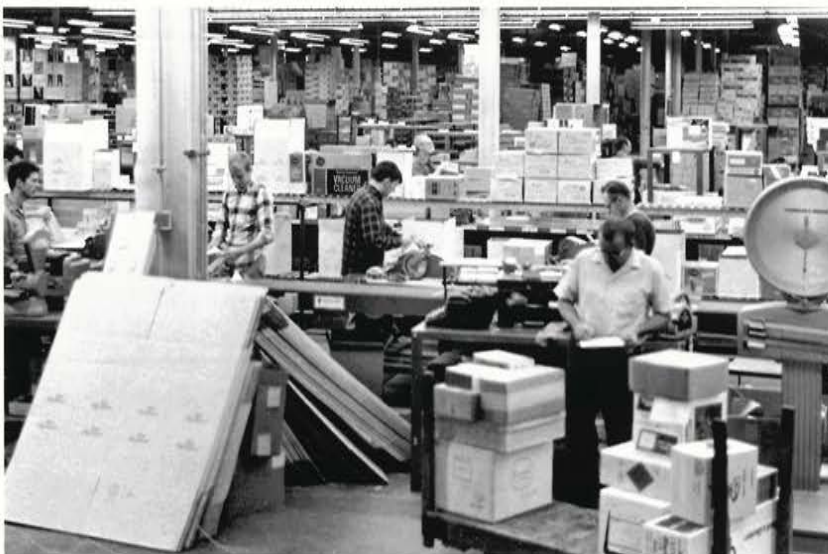
New Maritz Distribution Center opened in 1965 in Fenton.
