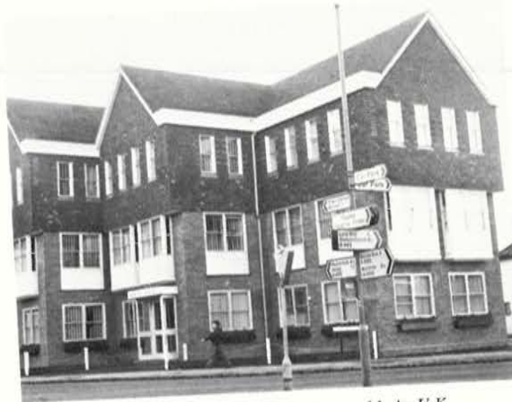
Maritz House, Marlow — Headquarters, Maritz U.K.
