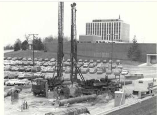
Construction of the new Travel headquarters building in 1985.
